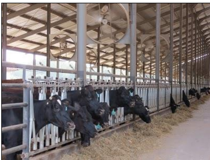
Figure 2. Fog ventilated dairy cattle housing at Ridiyagama national livestock development farm, which rare temperate breeds of dairy cattle.
